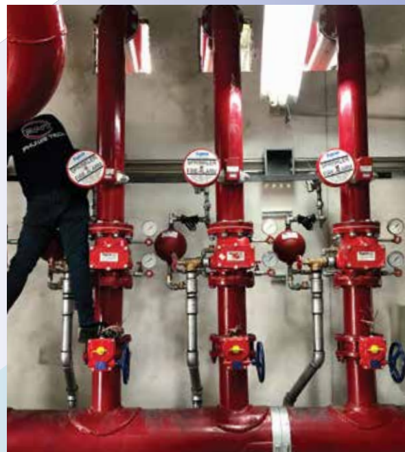
Fire Alarm System
